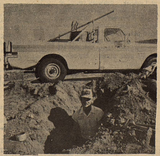
The foreman with Armstrong Mechanical is shown here installing water lines.
