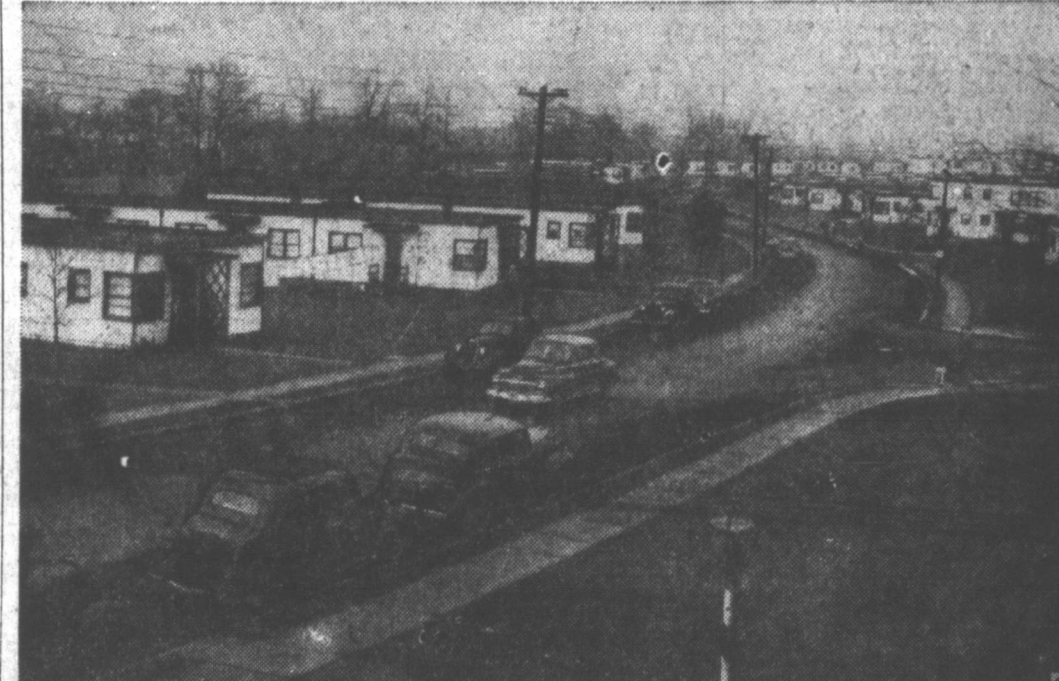
TOWNSPEOPLE BUY A COMMUNITY — Street in Winfield, N. J. 26 miles from New York, a community containing 700 houses which residents have voted to buy from the government for $1,550,000 through their own cooperative Mutual Housing Corporation.
