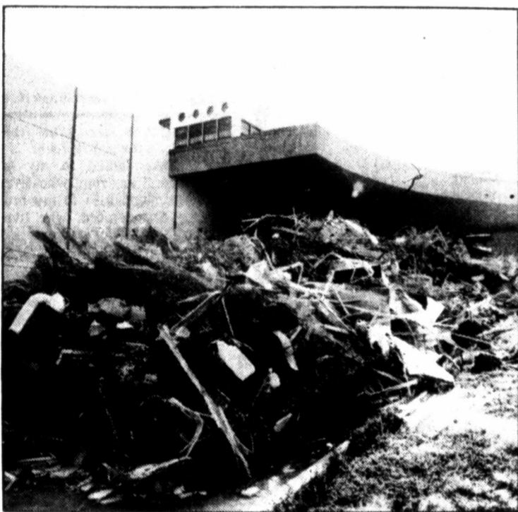
Mountains of refuse begin to pile up outside the old Highland General Hospital this week as demolition is
