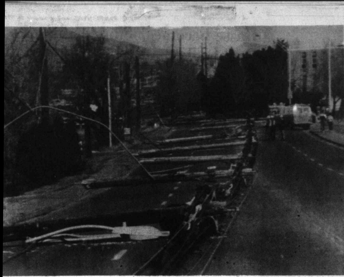
IN A ROW. Utility poles on 30th Street east of Denver, Colo., were toppled by high winds Sunday. Extensive damage occurred along the Colorado upper front range as Chinook winds developed gusts up to 137 mph Sunday resulting in extensive damage to numerous buildings. (AP Laserphoto)
