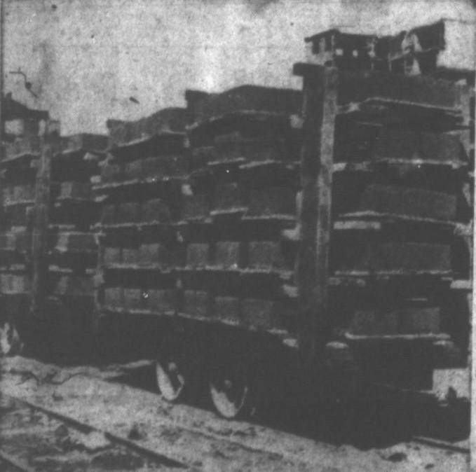
BRICKS FROM WAR'S RUBBLE —These bricks were made from the war rubble in Warsaw, Poland. In special mills located near devastated areas the rubble is ground, sorted, mixed into concrete and finally pressed into bricks. The bricks then go into the rebuilding of the ravaged city.
