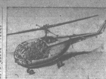
COMMUTER 'COPTER-This shows how a dozen passengers can be carried by the new feeder-liner helicopter developed by Bell Aircraft at its Buffalo, N. Y., plant. The craft, which cruises at 100 mph, is designed for rapid transportation between heavily populated and traffic-congested areas. In place of the 12 passengers, it can carry an equivalent weight of mail or cargo.
