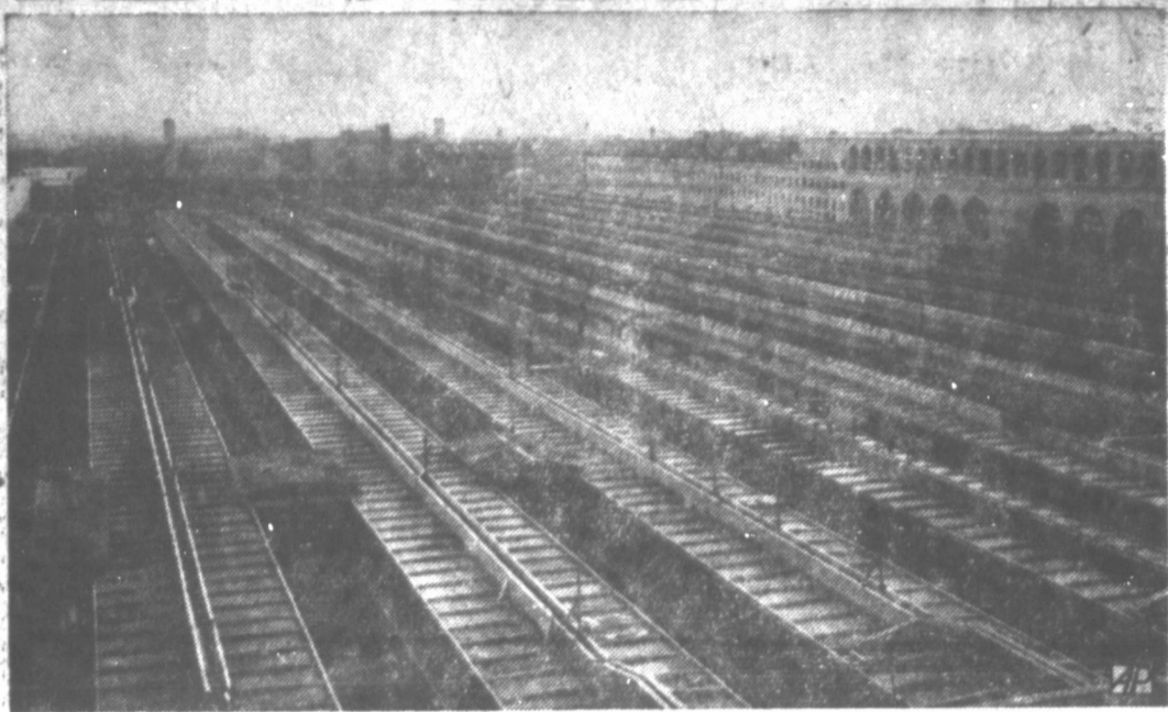
NEW GATEWAY TO ROME —Some platforms to serve railroad travelers in the new Central Station, Rome, Italy, will be usable in December but construction will continue into 1950.
