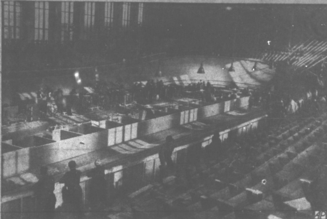
FOR BERLIN BIKE RACES — This new bicycle track of 10 1/2 laps to the mile was built in 14 days in West Berlin for the first of a series of six-day races in November.
