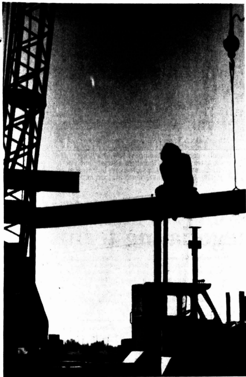
PROFESSIONAL OFFICE BUILDING construction is continuing, and plans call for the 12,500-square-foot building, located
