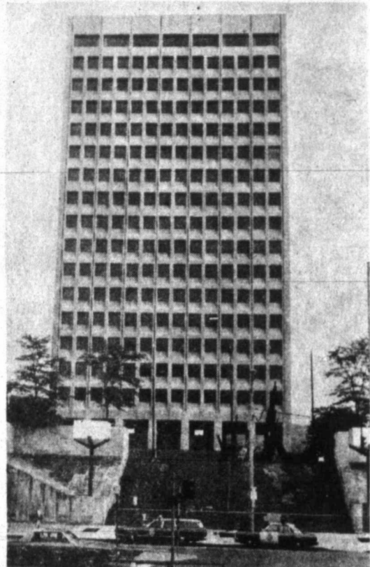
PCB-RIDDEN STATE office building in Binghampton, N.Y., is bound to prove expensive, even if the suits against the state fail. A total of $4 million has been spent since the fire on the building which cost $17 million.
