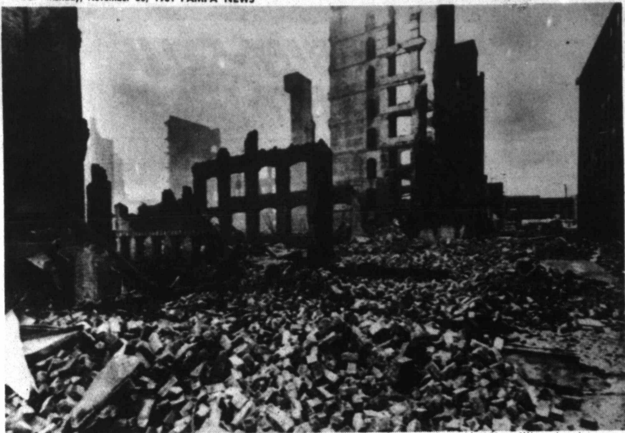
AFTER THE FIRE. The remains of some of the 17 buildings in Lynn, Mass., which were destroyed by flames early Saturday morning stand silhouetted against the Sunday dawn. The fire displaced nearly 750 people and caused an estimated $35 million in damages. Firefighters from 45 communities aided in battling the blaze which raged out of control for 16 hours. (AP Laserphoto)
