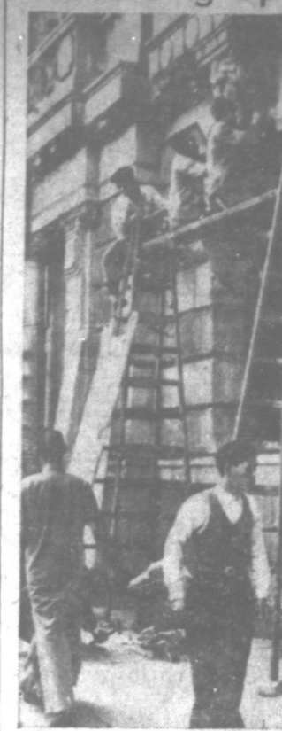
Chinese workers erect iron covers in front of the windows of the U. S. government-owned Glend Line Building, now the quarters of the U. S. Consulate in Shanghai. The besieged city feverishly prepared defenses as the Communists prepared to close a ring of men and guns around the metropolis.
