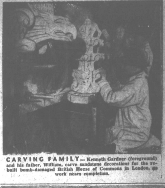
CARVING FAMILY —Kenneth Gardner (foreground) and his father, William, carve sandstone decorations for the rebuilt bomb-damaged British House of Commons in London, as work nears completion.
