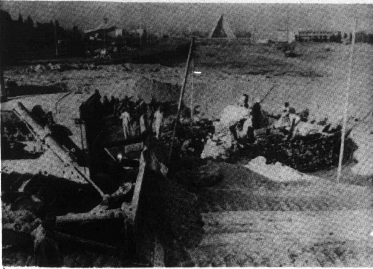
BURIAL SITE. Workmen build the mausoleum where Egyptian President Anwar Sadat will be buried on Saturday. The site is located one-half kilometer from assassination site. Tomb of the unknown soldier can be
