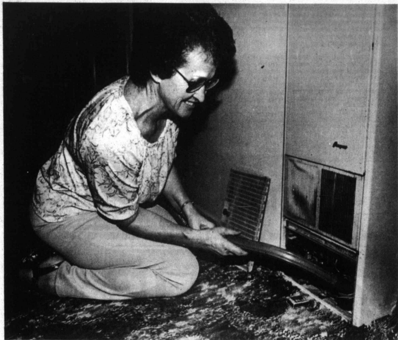
START CLEAN. Mrs. June Elliott of 1137 Sierra the summer can be a fire hazard, if not cleaned out before lighting the pilot.
