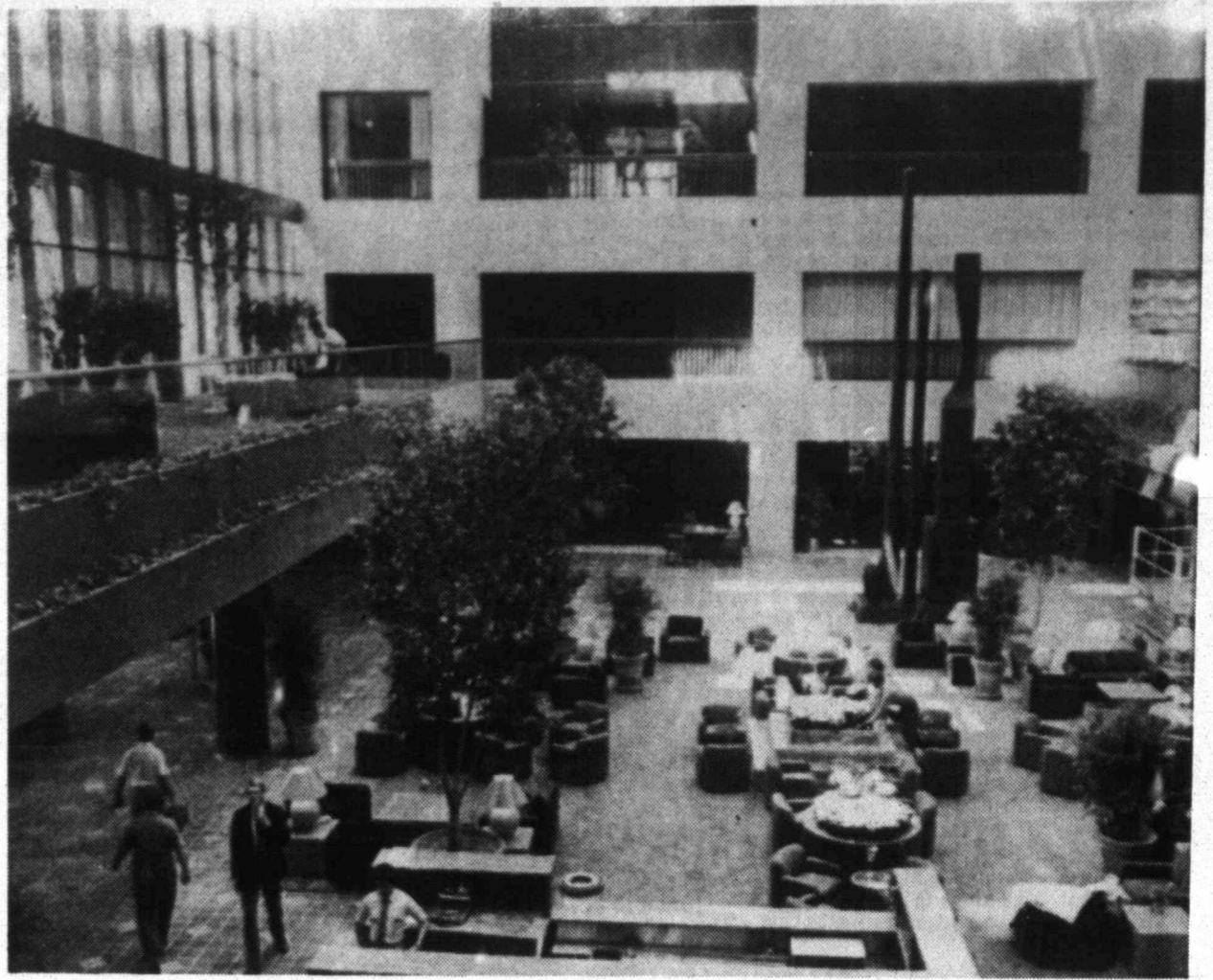
HYATT TO REOPEN. Hyatt Regency employees work in the lobby of the hotel Wednesday, preparing for today's reopening of the Kansas City Hyatt Regency. A new walkway spans the lobby at left in place of one of the catwalks that crashed onto a crowded dance floor last July 17, killing 113 people. The catwalk that remained was removed entirely. (AP Laserphoto)
