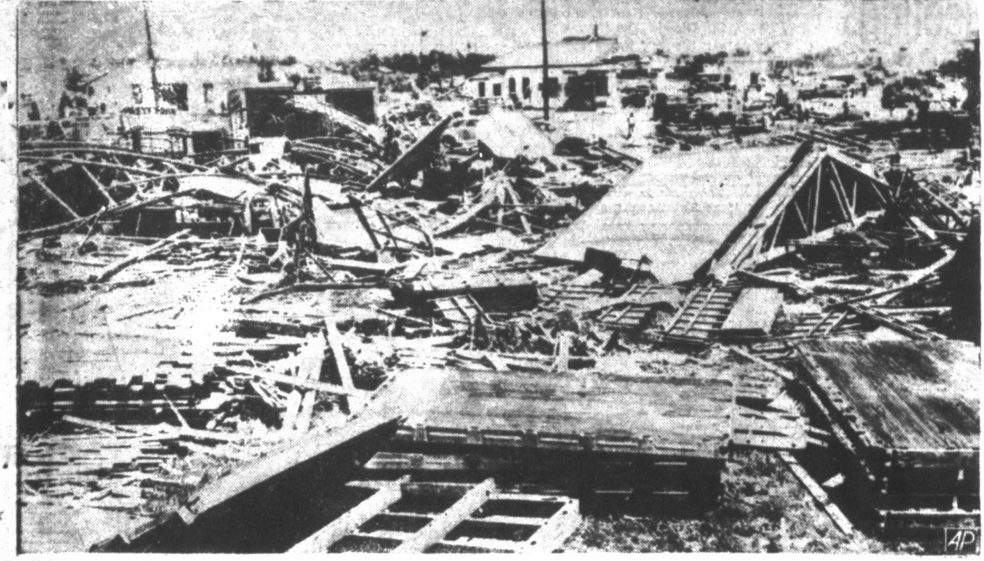
TEXAS TORNADO DAMAGE — Wreckage of the Lone Star Trailer Company and the Timberlock Body Company is scattered over a wide area after a tornado struck Amarillo. (AP Wirephoto)
