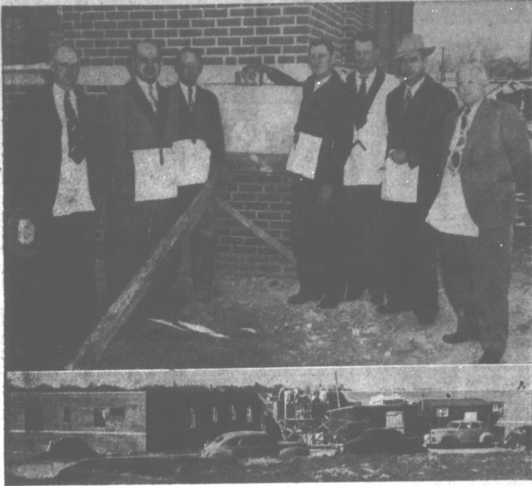
CORNERSTONE LAID —Laying the cornerstone for the new Hemphill County Memorial Hospital at Canadian this past week are (left to right) County Judge H. M. Wood, Tom Abraham, Logan Owens, Nick Morgan, Bob Whaley, John Wilkinson and Sam Allison. The ceremony was conducted by members of the Canadian Masonic Lodge. Lower picture is scene of the new building under construction. (Cut by courtesy of The Canadian Record)
