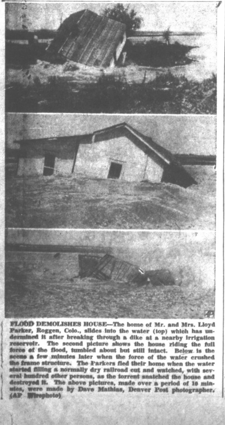
FLOOD DEMOLISHES HOUSE—The home of Mr. and Mrs. Lloyd Parker, Roggen, Colo., slides into the water (top) which has undermined it after breaking through a dike at a nearby irrigation reservoir. The second picture shows the house riding the full force of the flood, tumbled about but still intact. Below is the scene a few minutes later when the force of the water crushed the frame structure. The Parkers fled their home when the water started filling a normally dry railroad cut and watched, with several hundred other persons, as the torrent snatched the house and destroyed it. The above pictures, made over a period of 10 minutes, were made by Dave Mathias, Denver Post photographer. (AP Wirephoto)
