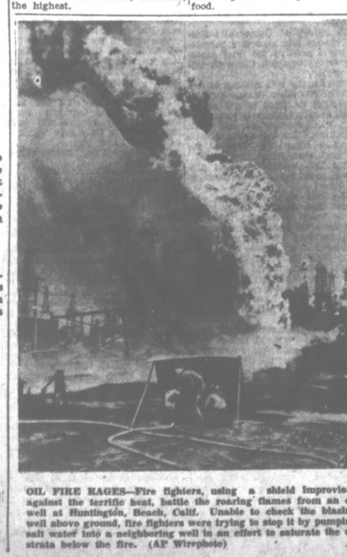
OIL FIRE RAGES — Fire fighters, using a shield improvised against the terrific heat, battle the roaring flames from an oil well at Huntington, Beach, Calif. Unable to check the blasting well above ground, fire fighters were trying to stop it by pumping salt water into a neighboring well in an effort to saturate the oil strata below the fire. (AP Wirephoto)
