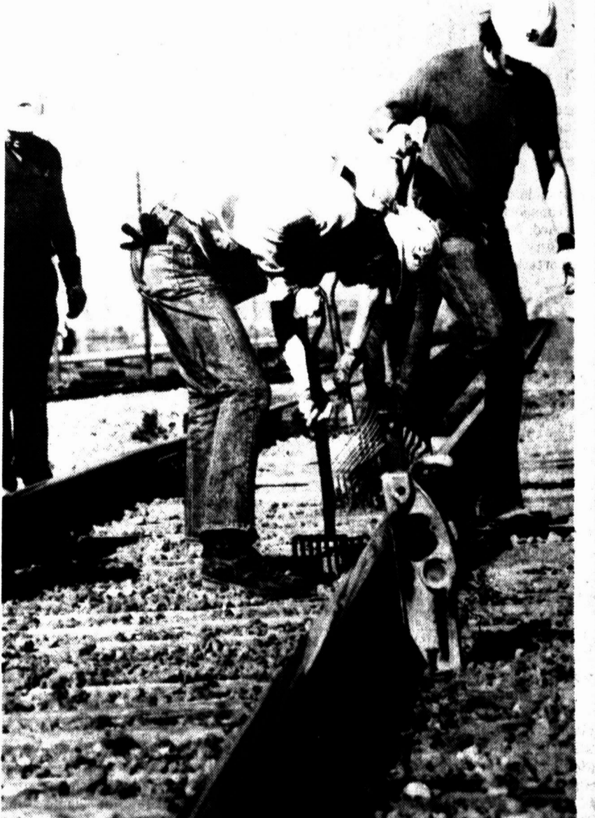
MODERN DAY GHANDY DANCERS working for the Santa Fe Railroad, are Scott Nix, left, Keith Lake, center, and Wayne Burnam. The men are repairing tracks near the Cabot Camp on Highway 60. Railroad repairmen travel along hundreds of miles of track checking conditions. (Staff Photo by Skyler Chapman)
