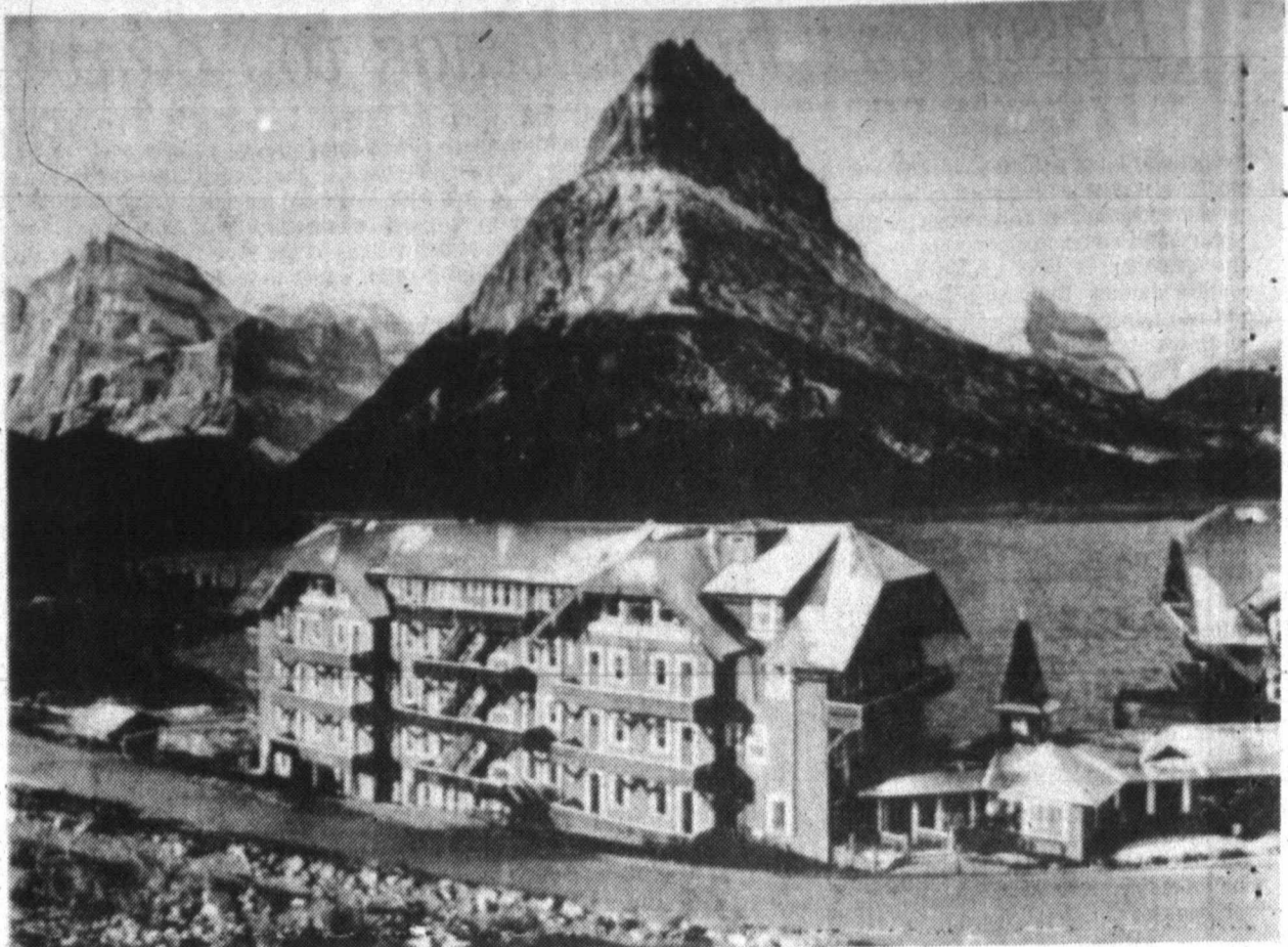
SPLENDID VIEW. Glacier National Park may be viewed from the windows of such hotels as the Many Glacier Hotel on Swiftcurrent Lake in Montana. More than 90 percent of the Glacier's rugged terrain is managed as wilderness, where human need are accorded secondary priority to those of animals residing there. (AP Laserphoto)
