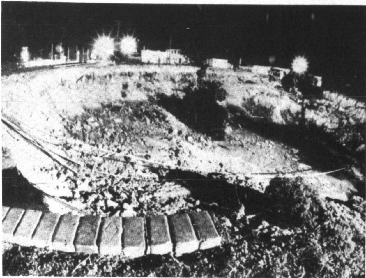
THE HOLE STORY. Bricks mark the remains of a wall at the edge of the sink hole in Winter Park, Fla., Tuesday night. Buildings in the background have been damaged by the hole, but the owners hope that the hole will not grow any larger. (AP Laserphoto)
