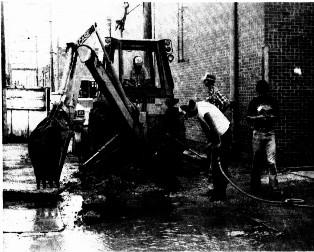
A BROKEN CITY water line in downtown Pampa early today had city employees John Smith, on jackhammer, and David Cook, right, working rapidly to pump water from several Southwestern Bell manholes. The water line break caused disruption of telephone service to 1,500 to 2,000 north Pampa residents today.
