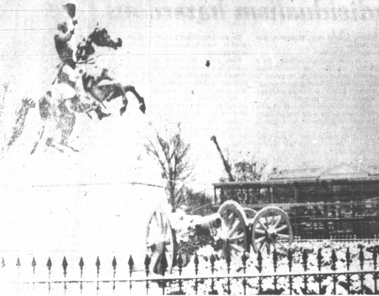
CAPITAL SCENE. The familiar scene of the White House scene of the White House framed by the Andrew Jackson statue in Lafayette Square in the foreground obstructed by the construction of a reviewing stand for the presidential inauguration Jan. 20. The nation's capital ushered in the new year with the first snow fall of the winter. In the background is the White House and the Washington Monument. (AP Laserphoto)
