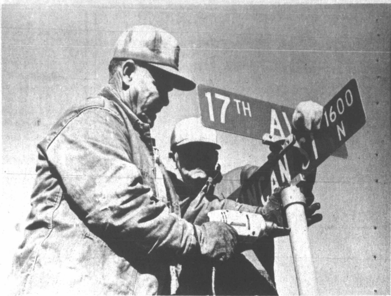
NEW SIGNS are replacing the rusty, vandalized signs marking intersections throughout the city. City street department employees, J. C. Clennault, left, and Floyd Smith, right, place a reflectorized sign at
