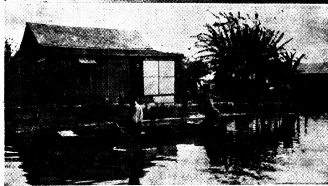
Water washes over highway on eastern edge of Eastland, Texas, (top photo) after heavy rains brought creeks out of their banks. In the bottom photo Joseph White arrives home via boat as floor waters surround his Brownwood, Texas, home and rise to within a few blocks of county court house.
