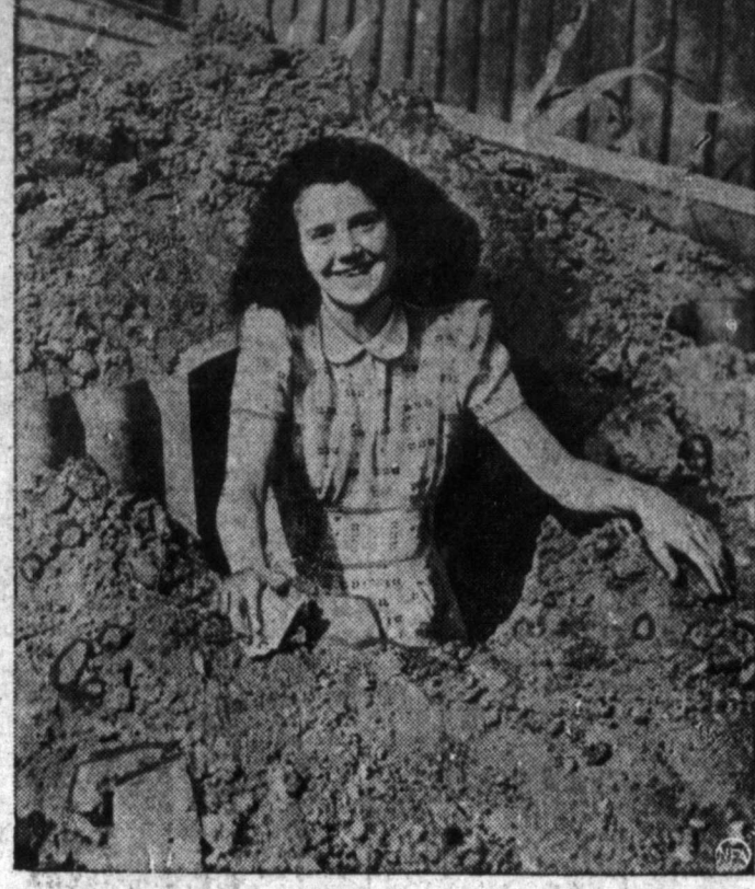
A Nazi bomb wrecked her home, blasted most of the earth covering off the the family air
