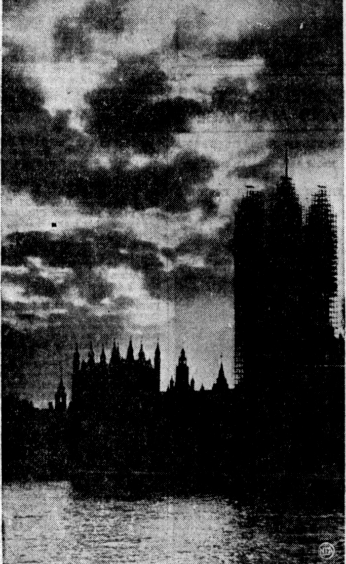
Not a new skyscraper going up, but an ancient cathedral, protected against bombing. This beautiful yet grim silhouette at sunset is presented by the protecting scaffolds thrown around the towers of London's famed Westminster Abbey.
