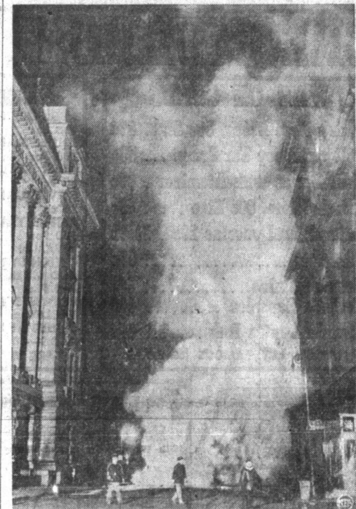
You're wrong. It's not a picture of a bombed European city, but a New York street scene. This geyser of steam shot up in the heart of the financial district, when a steam pipe under the street burst.
