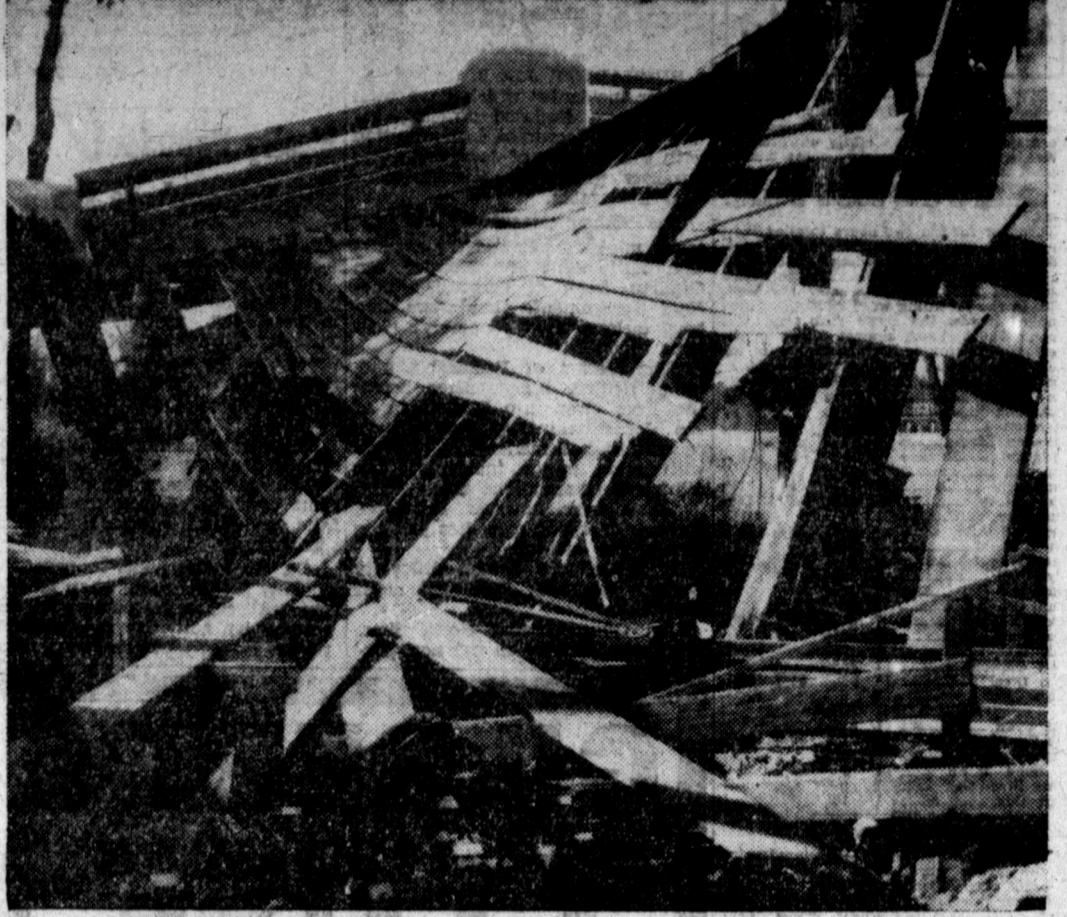
Forty persons were injured when a section of boardwalk collapsed while a large crowd was watching a fireworks display at Ft. Worth, Texas. Only 15 persons were required to remain in the hospital for more than examination. Officials believe that recent heavy rains, weakened supports beneath the walk and the weight of the crowd proved too great.
