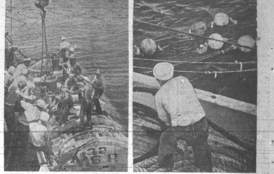
The sunken submarine Squalus, undersea tomb of 26 U. S. Navy men, will be floated from the bottom of the Atlantic off Portsmouth, N. H., by seven giant pontoons. Shown at left, above, is one of them, with seaman of the rescue ship Falcon attaching "comealongs". To each comealong will be fastened giant lifting chains. Air hoses attached to the Squalus are kept clear of the Falcon by the globular floats shown at right.
