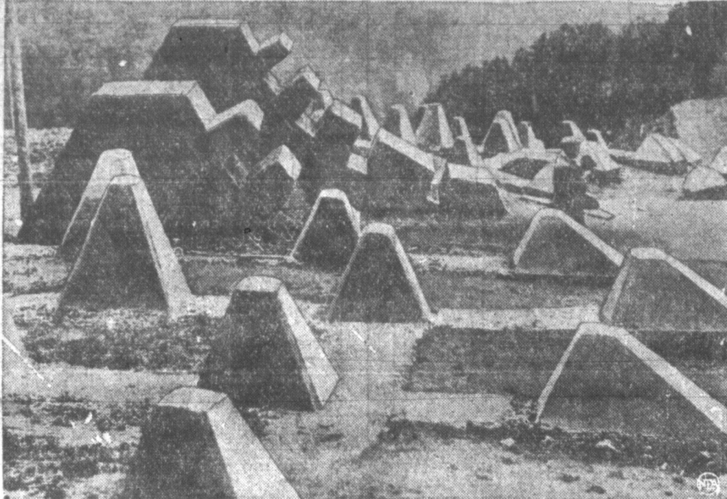
These might slabs of steel and concrete have all the appearance of ruins left by some vanished prehistoric race. Actually they are tank barriers along the Siefried Line by which Germany hopes to hold French tanks in check if war comes. This picture was flown across the Atlantic to NEA Service and The Pampa News.
