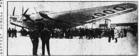
Germany's latest bid for leadership in airplane design is the giant machine shown here—the largest land plane in the world. It is a Lufthansa Junkers, recently completed and sent on a test flight to Croyden Airport, England, where you see her here. The G-38, as it is called. is powered by four motors. Quar-ters for 14 passengers and a crew of six occupy part of the leading edge of the extremely thick wing where it meets the fuselage.
