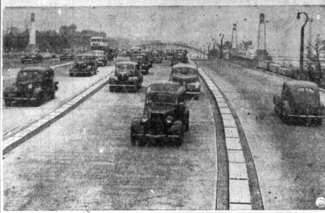
Traffic lanes, "made to order" by curbs that rise and descend, are helping solve traffic problems along Chicago's lake front highway. Curbs are normally flush with the pavement. Hydraulic lift quickly raises them nine inches, making various combinations of lanes in the roadways, depending on traffic volume of the moment. The new elevating curbs, pictured above in use, were designed by traffic engineer Otto E. Jelonek.
