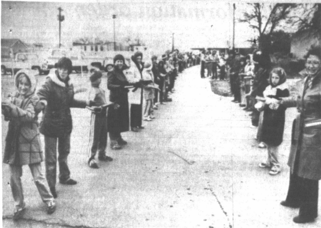
MOVING DAY. One book at a time, a 1,000-member chain moved about 24,000 volumes into the new library in Yukon, Okla., Saturday. Books were moved two blocks from the old facility to the new one
