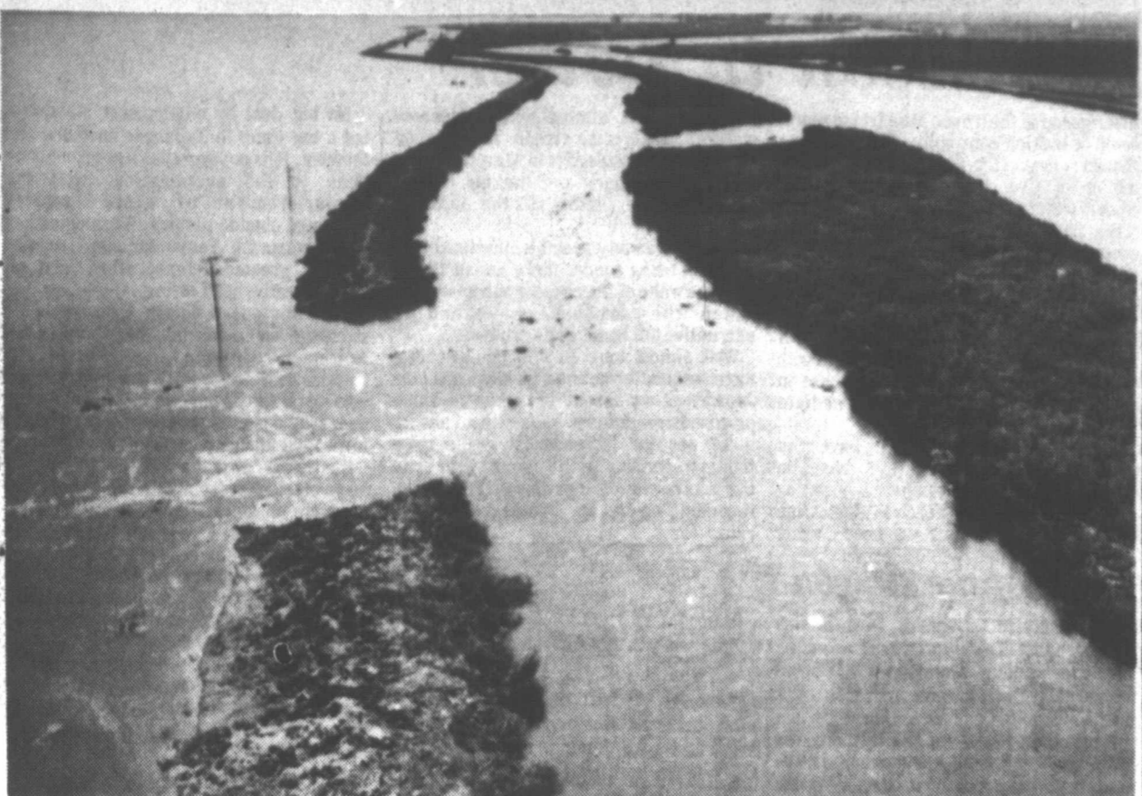
RESEMBLING THE MISSISSIPPI DELTA COUNTRY, this San Joaquin Valley scene shows the damage and flooding of the countryside near Stockton, Calif. A levee leak, attributed to a busy beaver in the Lower Jones Tract, chased 200 families
