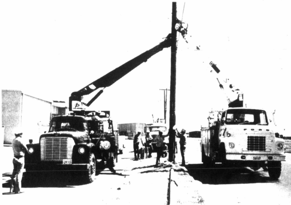
QUICK WORK by four Southwestern Public Service crews resulted in the return of electrical power to the Coronado Shopping Center within eight hours
