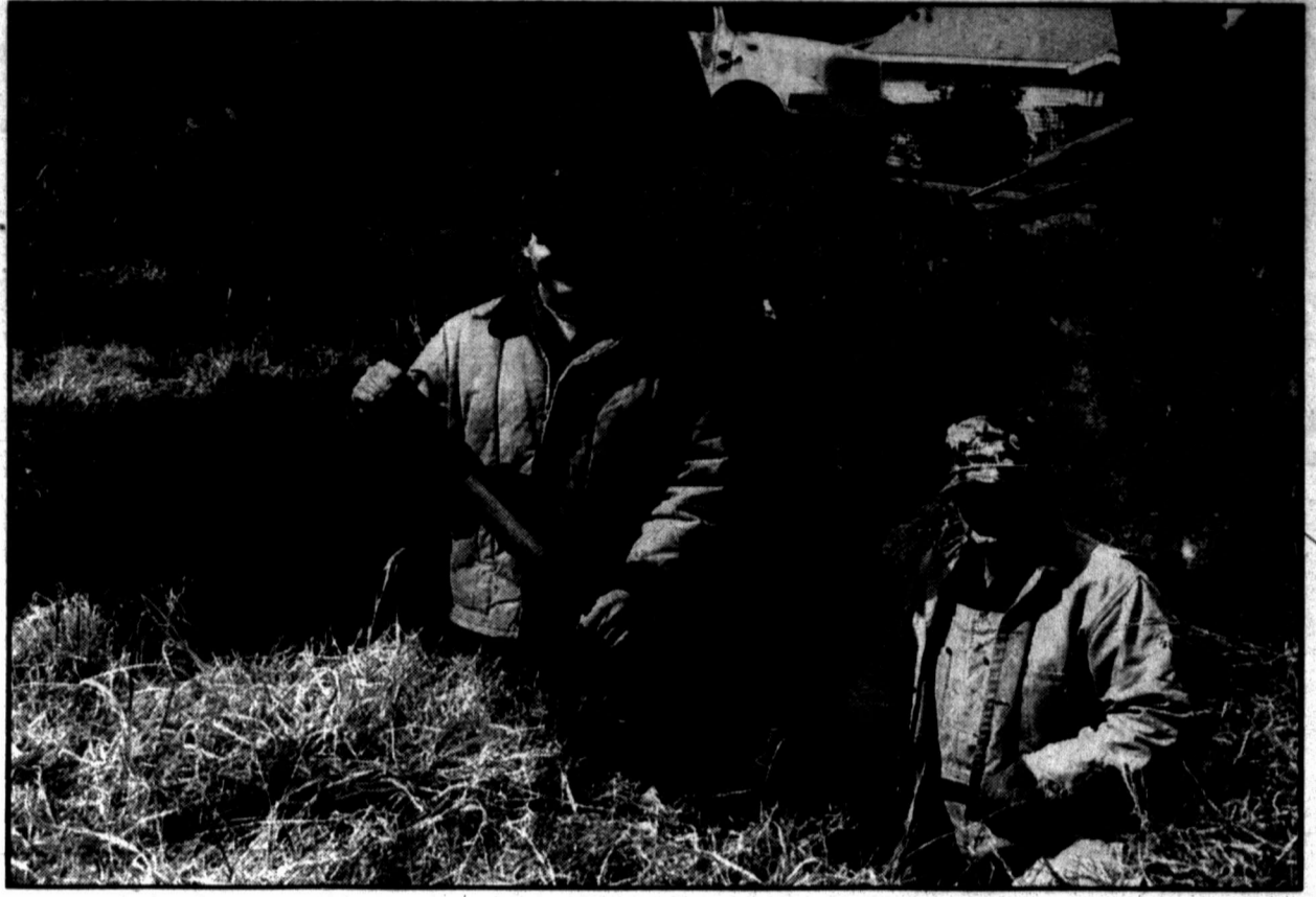
(Pampa News photo by Darlene Holmes) Dave Carter and Preston Pairsh, both of Pampa, find themselves digging a hole Monday. The two men were busy repairing a gas leak that had developed in the 300 block of East Browning.
