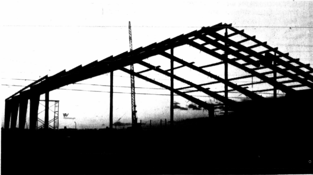
DUSK FALLS OVER STEEL BEAMS in construction of the Pampa Youth and Community Center. The $375,000 expansion was begun in February and promises a 25,000 square foot addition that will house a racketball court, an indoor jogging
