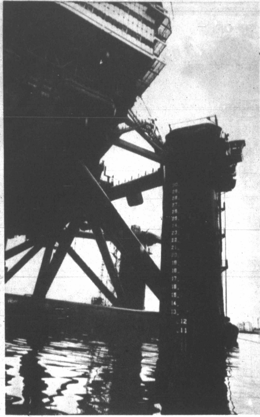
LOOK ALIKE. This close up shows a good view of the legs of the "Henrik Ibsen", accomodation platform, sister rig of the capsized "Alexander Kielland". This photo shows the portion of the doomed platform which broke, causing the loss of over 100 men.
