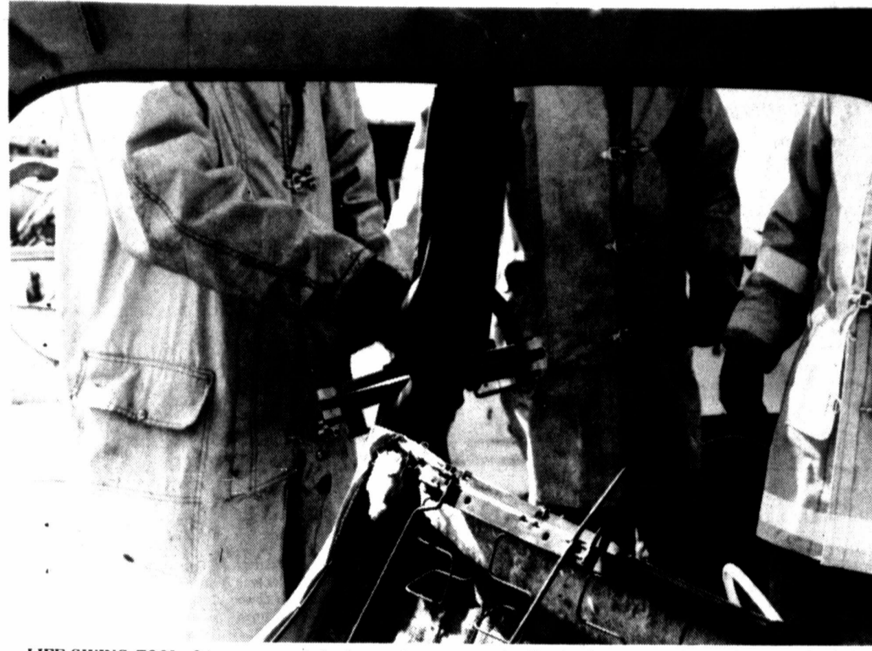
LIFE-GIVING TOOL. It's a scary sight from the inside, but for those trapped in autos after an accident — it could mean life. Members of the Pampa Fire Department are practicing using the new Hurst "Jaws of Life" rescue tool recently received by the department. Crews from each of the three stations will spend time at a local auto salvage yard this week learning effective use of the tool in the event it is needed for future rescue efforts. (Photo by Larry Cross)
