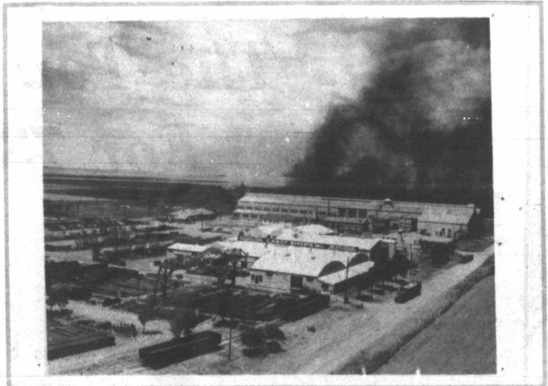
Early photo of Machinery Division when production of pumping units was at its height. This production was phased out in 1966, and manufacture of mobile hoist rigs was beginning to emerge in importance at Machinery Division
