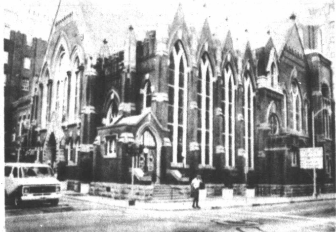
THE FIRST BAPTIST CHURCH of Dallas is the largest Southern Baptist Church in the world. Located in downtown Dallas, the church is funded entirely by contributions from its 20,000-plus members, who give to the church in a spectacular service every year. (AP Laserphoto)
