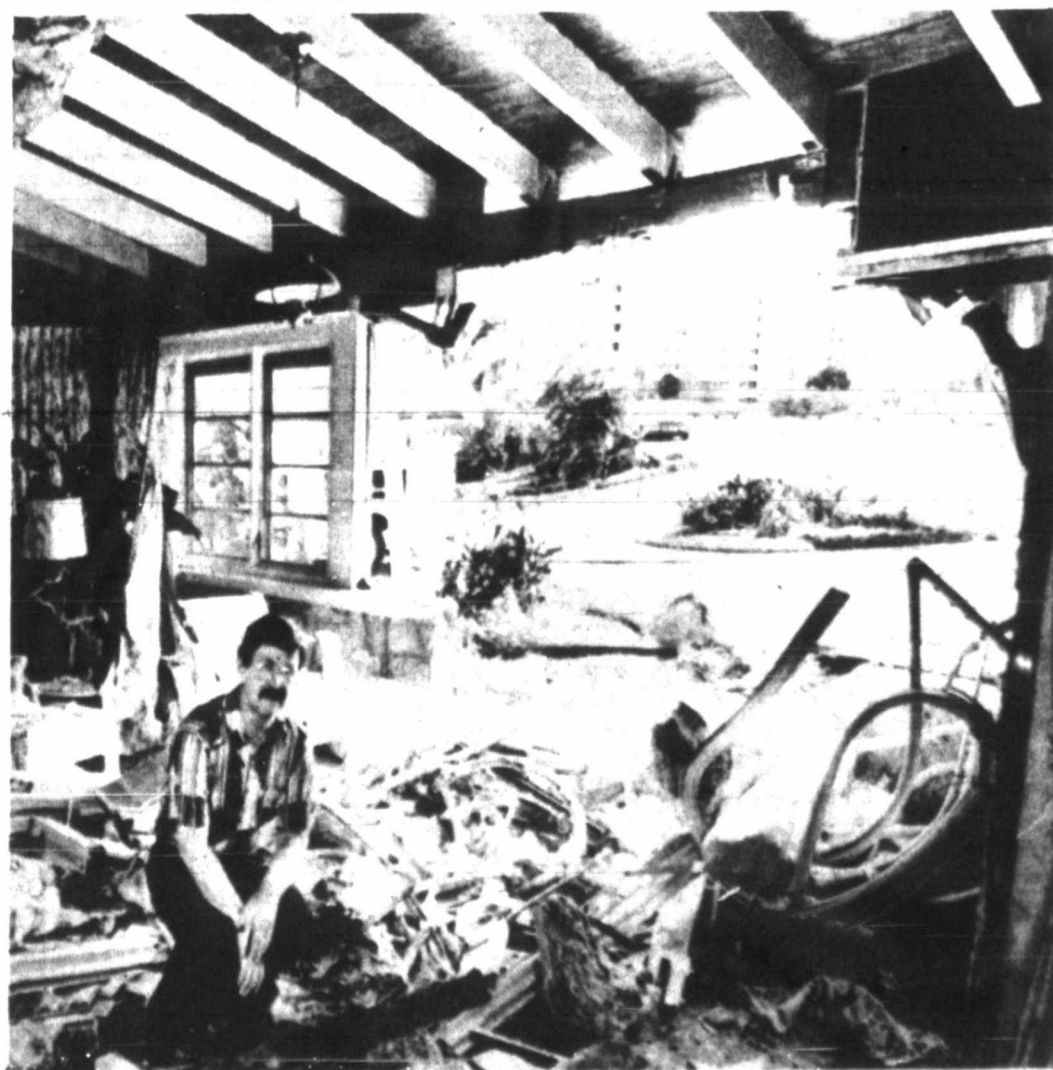
JACK STARBUCK sits in his living room and examines the wreckage caused Sunday morning when 22-year-old Ardy Bernstein plowed through the front wall of Starbuck's home after losing control of his sports car. Bernstein suffered two broken legs, but Starbuck was not injured.
