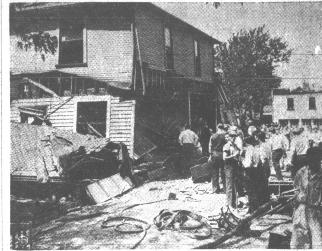
When explosion rocked this temporary frame school building at Barberton, Ohio, more than 50 school children were injured. Four perhaps fatally. Blast, believed to have been caused by leaking gas, blew walls from structure and buckled floors. In foreground is one of many desks hurled out of building.
