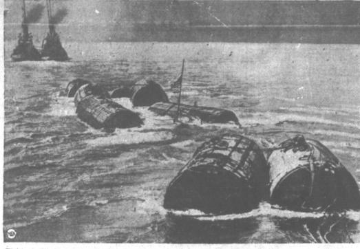
Eight air-filled pontoons, having lifted submarine Squalus, will keep ship affoat as it is towed to port. Picture shows S-51, which sank in fall of 1925, being pulled homeward after it was salvaged in spring of 1926. Flag at half-staff indicates submarine's position—directly below surface.
