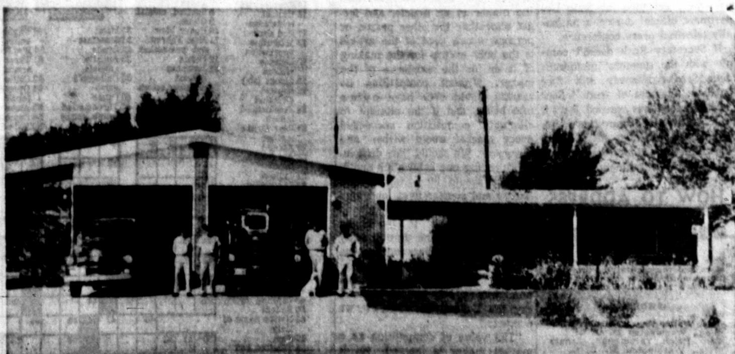
FIRE STATION NUMBER 2 at 1010 S. Barnes. This station has 3 firemen on duty at all times. It is equipped with one 750 Broadman Pumper with 400 gallon booster tank, and a booster truck with 200 gallon tank.
