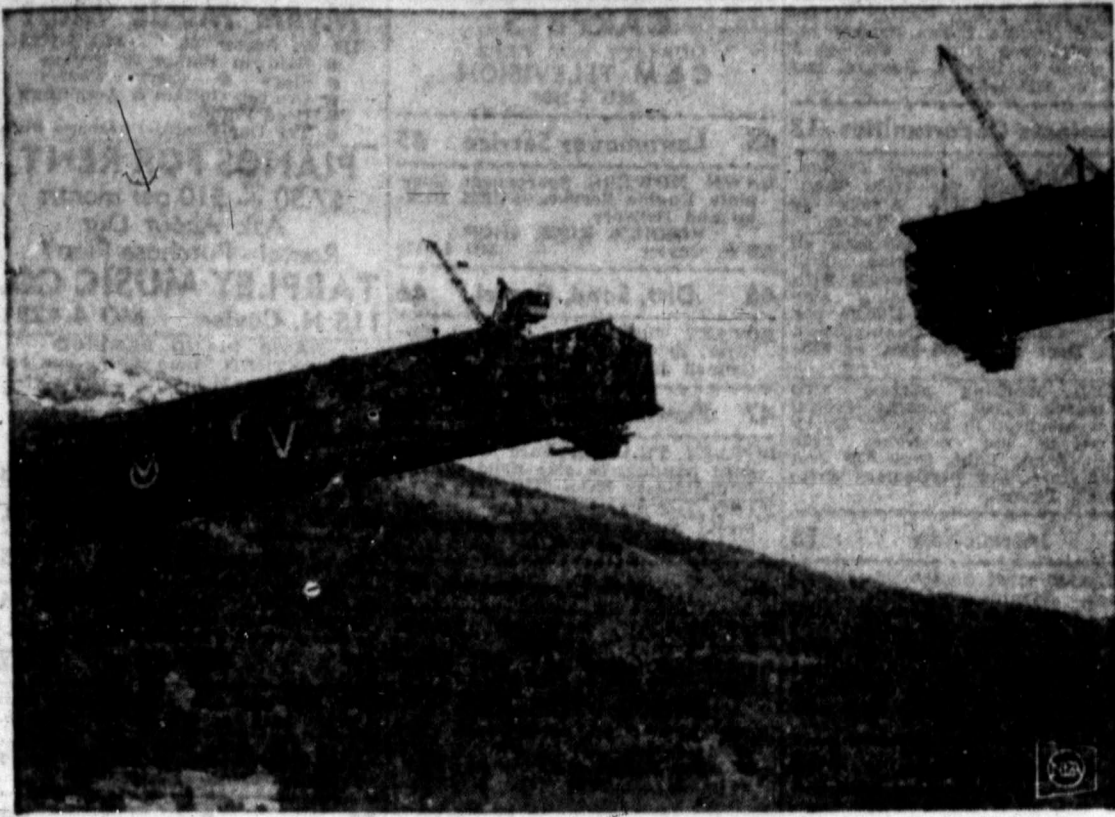
BRIDGING SPACE AND TIME —Just as America is engaged in a massive highway building program—the 41,000-mile Interstate System—so has Europe embarked on a similar effort. As economic barriers between nations come down, superhighways, tunnels and bridges conquer physical barriers. An example is the giant Europa Bridge over the Sill Valley in Austria, shown above as the last gap in its 2,700-foot length was being closed. The bridge is 625 feet high at this point. It will provide a faster link between Innsbruck and the Brenner Pass.
