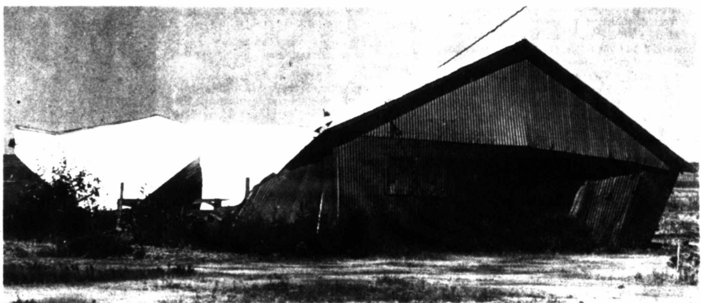
Storm damages barn
